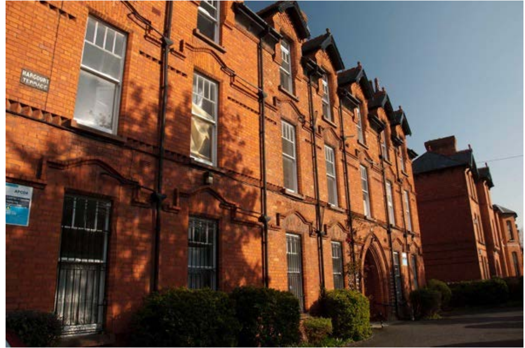
Former Broadstone Studios at Harcourt Terrace
